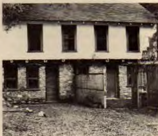
New Zendo will be in this building, with sleeping upstairs
